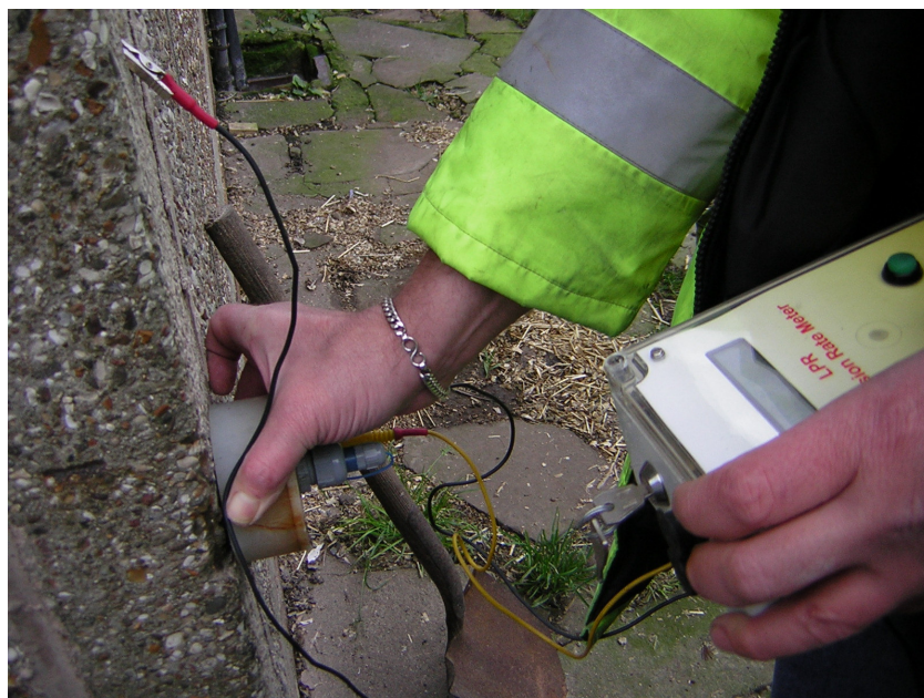
Photograph 4 – Linear Polarisation Corrosion Rate Monitoring
